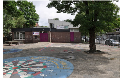
De Kameleon School in Rotterdam
